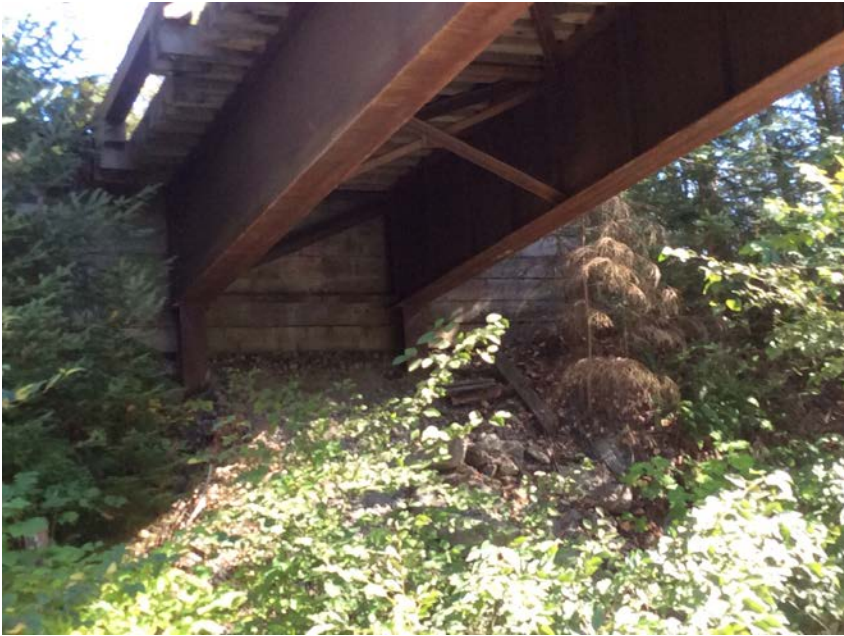
Left Bank Abutment when facing downstream
