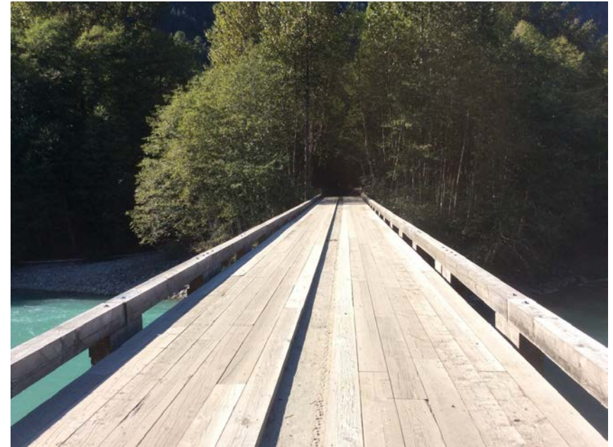
Right approach viewed from bridge
