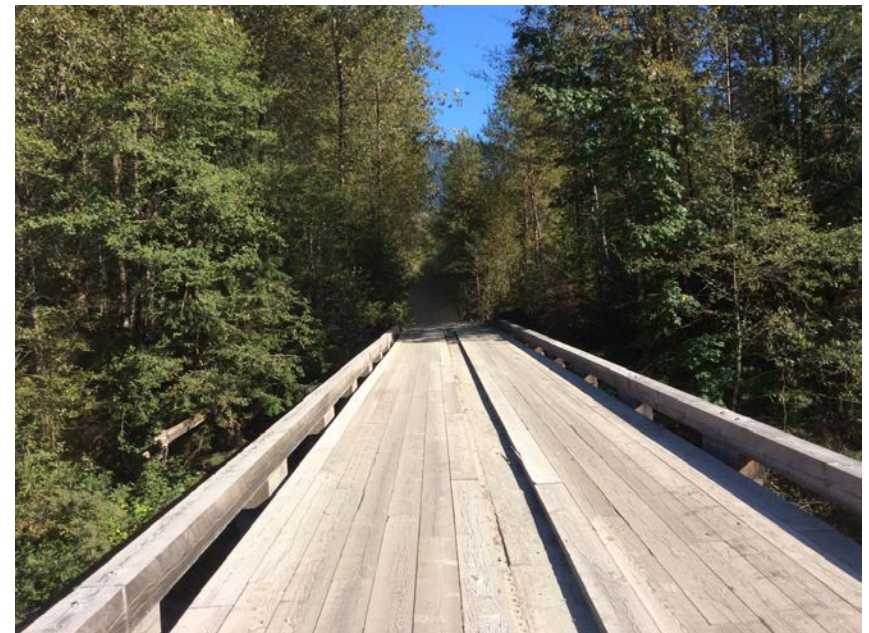
Left approach viewed from bridge
