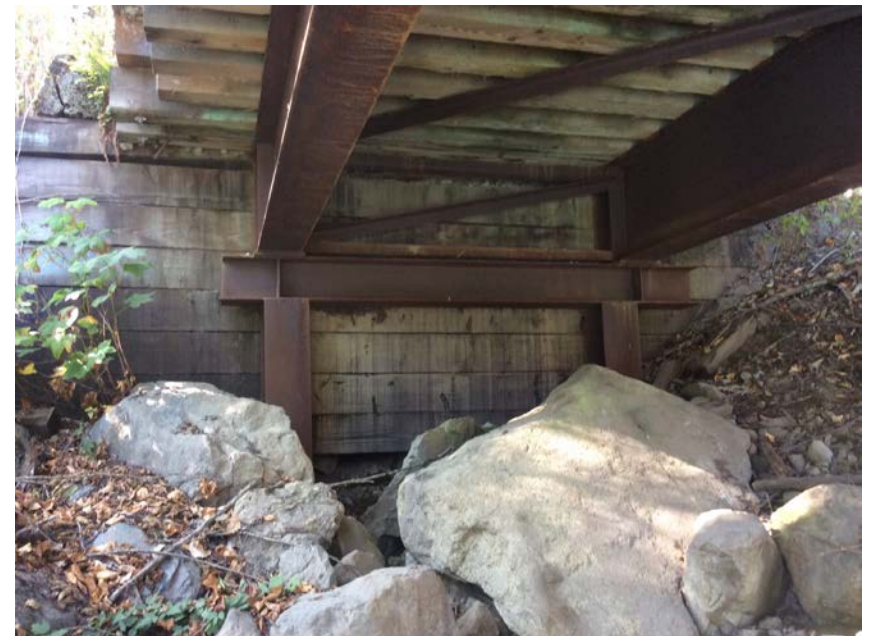
Right Bank Abutment when facing downstream
